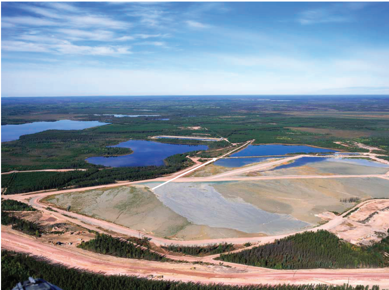
FIGURE 6.1 Tailings management area at Cluff Lake in 1999, Saskatchewan, Canada. The tailings are held behind an earthen dam. SOURCE: AREVA Resources Canada, Inc.
