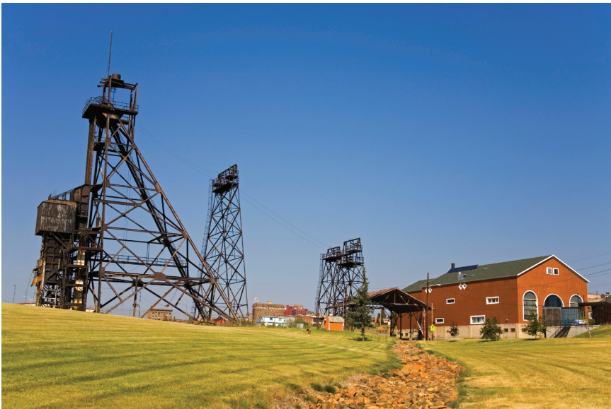
FIGURE NS.6 Underground mine head frame and hoist room. SOURCE: Courtesy Richard Cummins/SuperStock.
