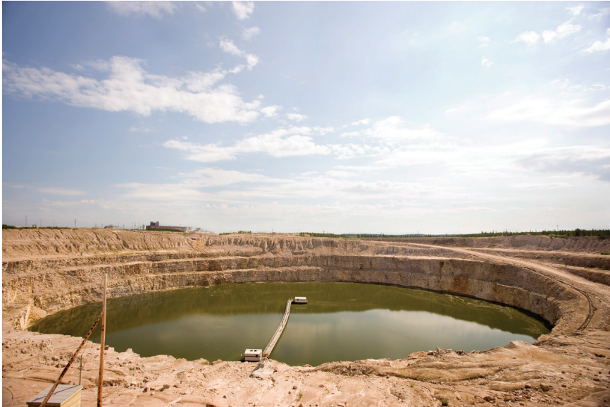
FIGURE 6.2 Waste management in the JEB pit at McClean Lake in Saskatchewan, Canada. SOURCE: AREVA Resources Canada Inc.
